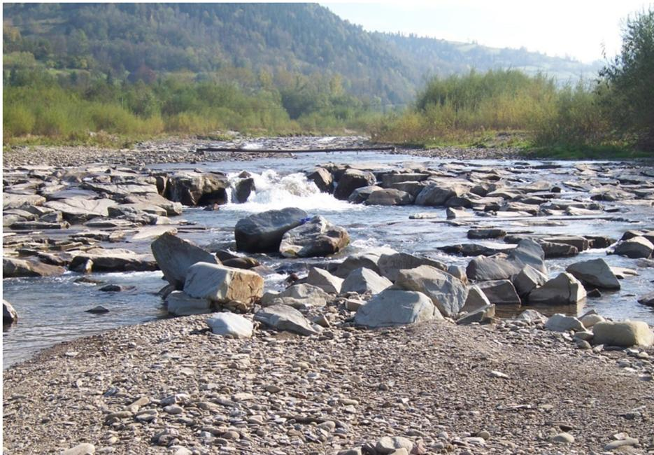
**Fig. 5.** Sloping apron of the block ramp, damaged as a results of the freshet wave
