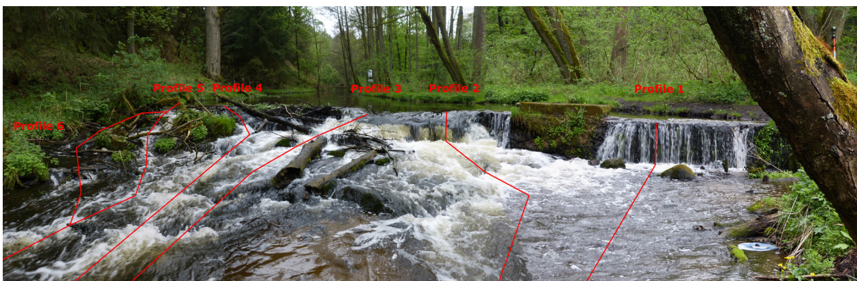
Fig. 2. Hydraulic structures with marked profiles (photo by K. Plesiński)
