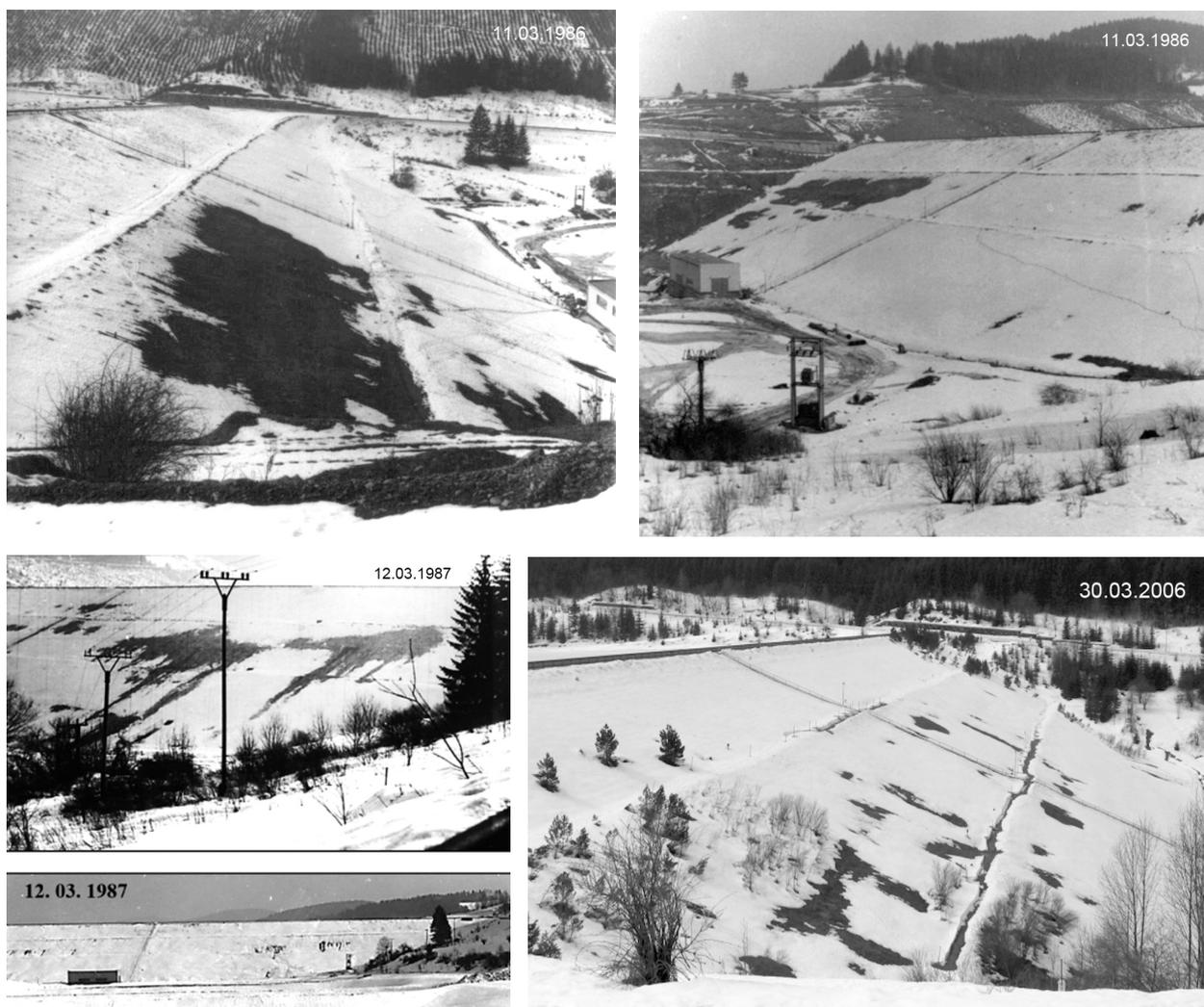
**Fig. 3.** Karolinka VD – seepage on the downstream face of the dam (archival photographs by PM and VD TBD)
