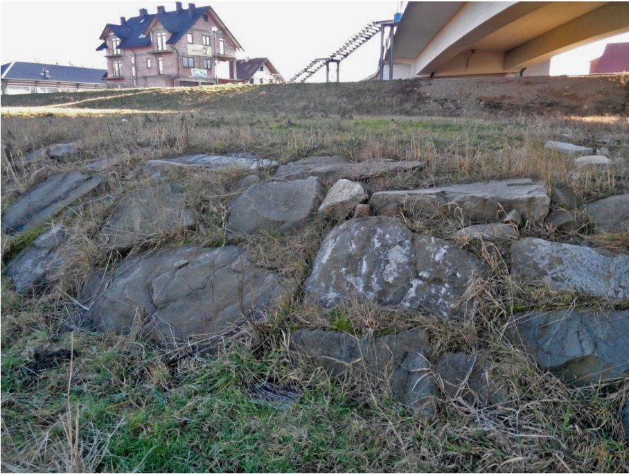
Fig. 5. Stone rip-rap in the first studied point (Nowy Targ on the Czarny Dunajec River)
