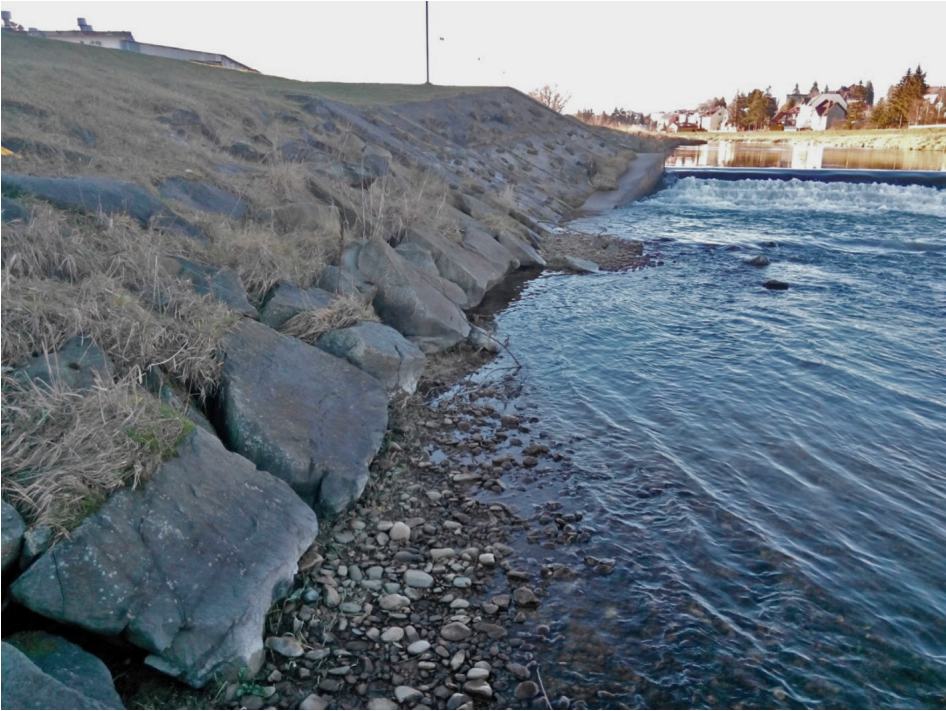
Fig. 6. Stone rip-rap in the second studied point (Nowy Targ on the Czarny Dunajec River)
