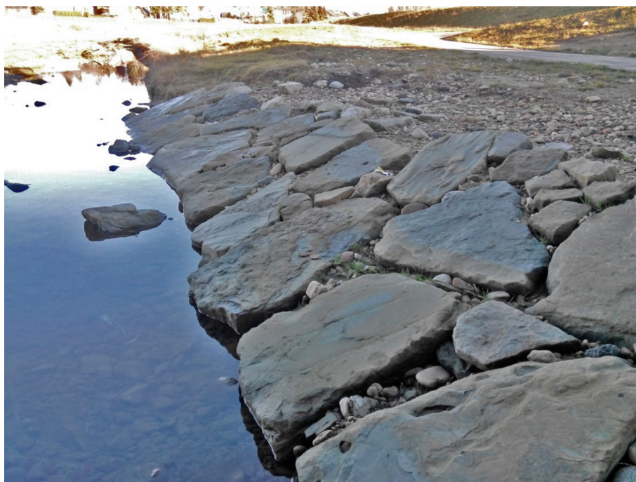
Fig. 7. Stone rip-rap in the third studied point (Nowy Targ on the Czarny Dunajec River)
