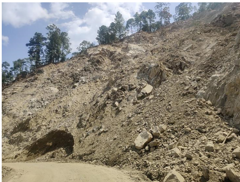
Fig. 2. Field photographs of landslide activities in Tanakpur block (Photo by the authors)
